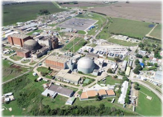
ATUCHA 1 First nuclear power plant in Latin America (362 Mwe) ATUCHA 2 Commissioning in 2014 (745 Mwe)
