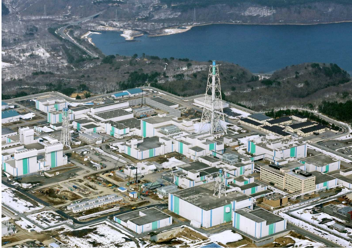
The troublesome Nuclear Fuel Reprocessing Plant in Rokkasho, Aomori Prefecture
