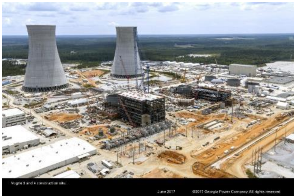
Figure 15: Vogtle 3 & 4 under construction[74]
