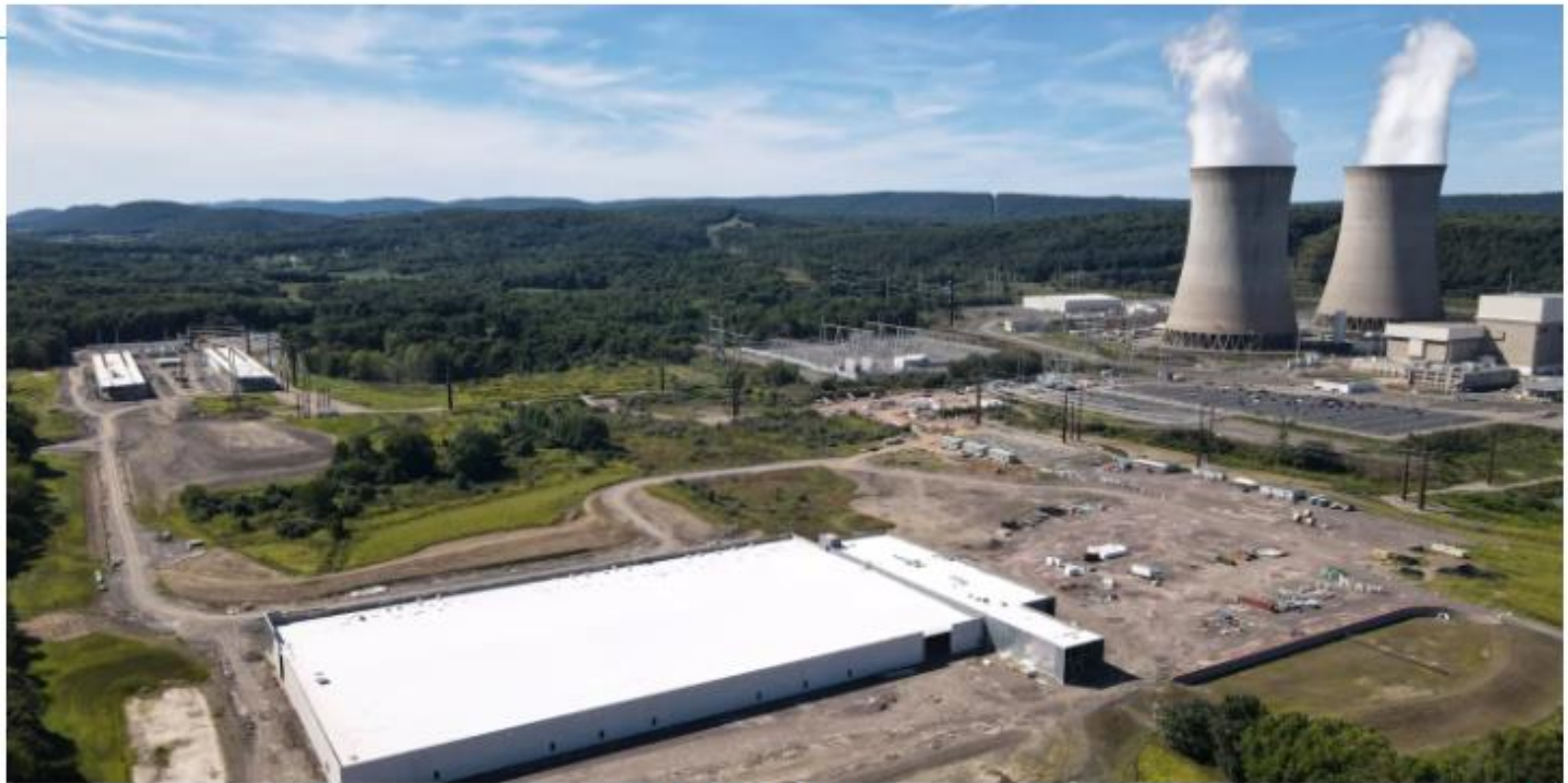
Photo: Talen Energy
