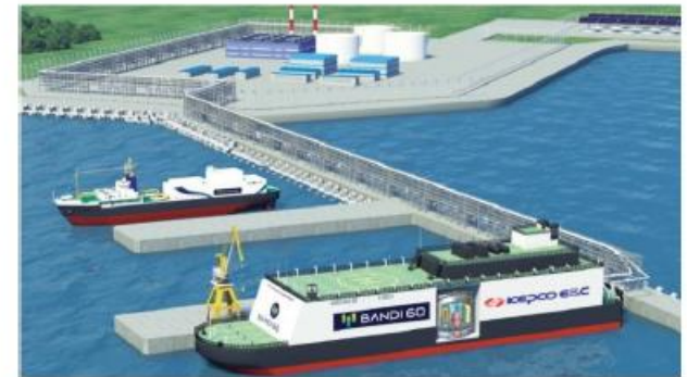
A floating nuclear power plant based on the BANDI-60 reactor (Image: Kepco ESC)
